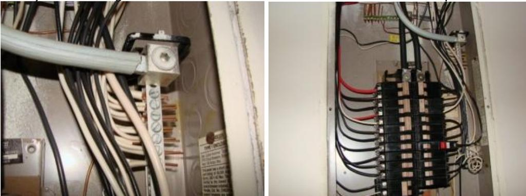
2). The well pump 12 gauge conductors are over-fused and enter a 30 amp double pole circuit breaker inside the main panel.
