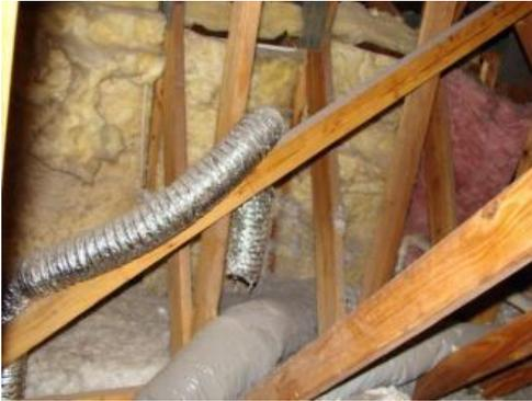
Recommend a fully qualified licensed contractor replace the flexible duct with smooth metal ducts and terminate the ducts up through the roof inside a damper type dryer vent hood with out screens.
